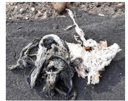
Shredded tampons pulled from pump at Lift Station 6.
