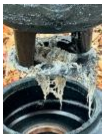
Flushable Wipes hanging from pump
